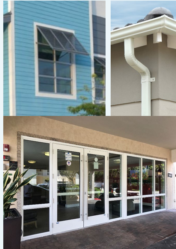
WHITE METAL FINISH AROUND STOREFRONT, LOUVERS AND GUTTERS
